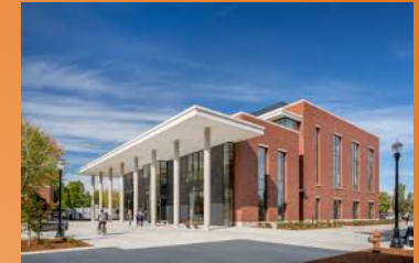
Figure 6. Johnson Hall at Oregon State University. LLE unit installed in John 214.
